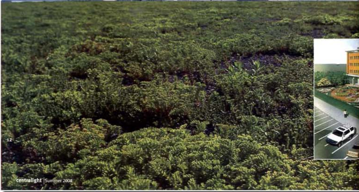
Sedum like this will be planted on more than half of CMU's Education Building roof by Xero Flor, the company that installed the green roof on the Ford Dearborn Truck Assembly Plant shown here. Inset: a sketch of the Education Building.
